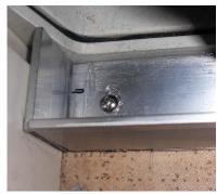
accommodate the two C" thick end caps.) The aluminum cuts easily with a hacksaw or other metal cutting tool. Slide one side of an end cap under each end of the long piece of angle bar as shown in the photo to the right. Then cut the flat bar to fill in the empty space under the angle bar between the two end caps. Drill through the angle bar and
