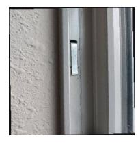
Identify the take-out clips: Find the small metal take-out clips located in the side jambs, just above the lower sliding sash. There are clips on both sides of the window.
