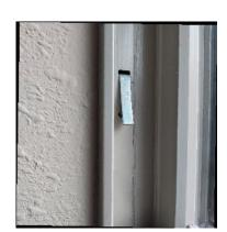
Remove the sash: Pull the sash toward the interior of the room and remove it from the frame.
